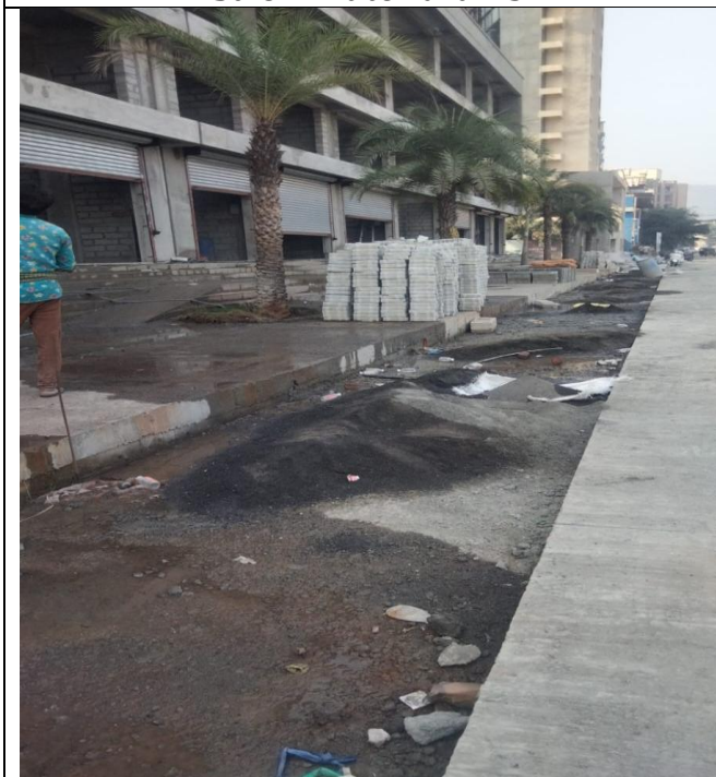
Strom water drains
