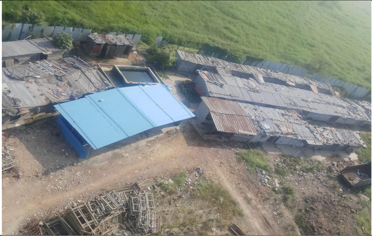
Labour Camp on Site
